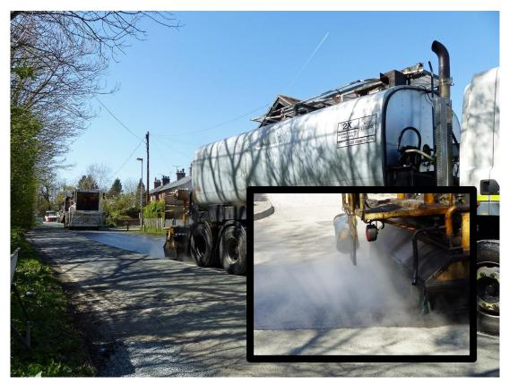
First a layer of hot liquid bitumen (known as binder) is applied to the road surface
