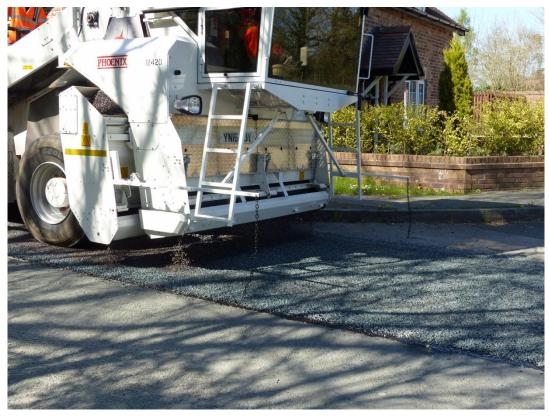
Then 6mm loose chipping were put on top – to fill in the gaps – this is called 'racked' surface dressing. Techniques used do vary.
