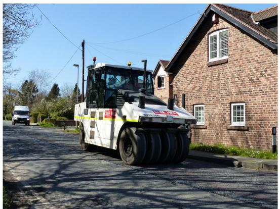
The loose chippings are then rolled to embed them into the layer of bitumen to make a strong surface. Vehicles driving on the road will continue this process.
