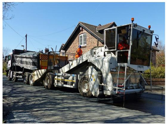
Straightaway loose chipping are put on top of the layer of bitumen. In these works in Kinnerton Road near Chester, 10mm chippings were applied first.
