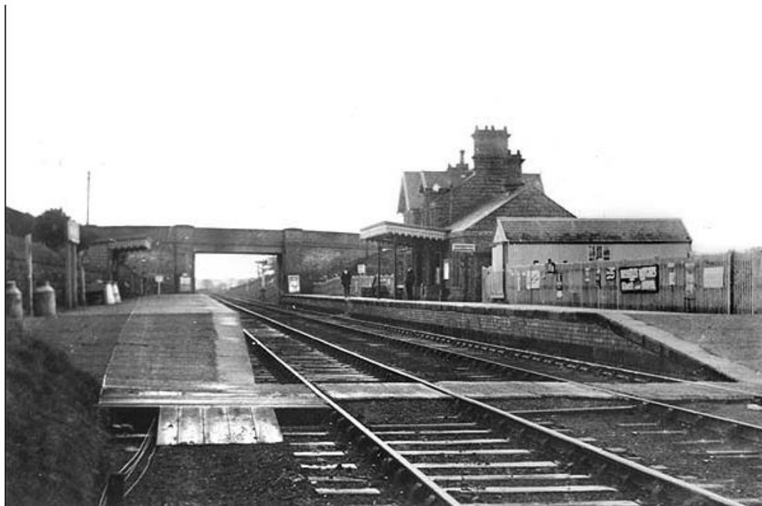
Malpas Station looking south
