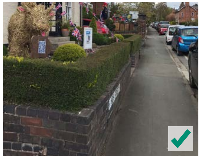
Figure 70: Red brick and hedgerow boundary treatment on High Street
