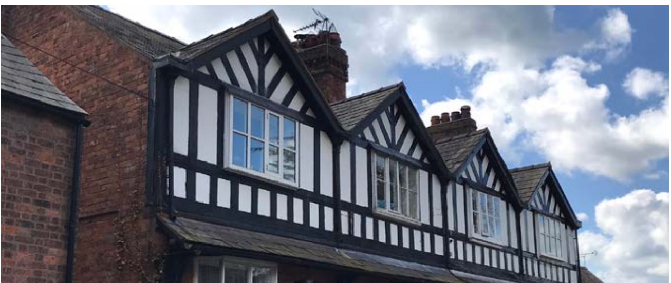
Figure 97: The use of black timber frames (particularly on gable ends) and pale render form part of the local vernacular and should therefore be represented in new development.
