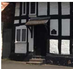
Timber frame single pitched overdoor canopy
