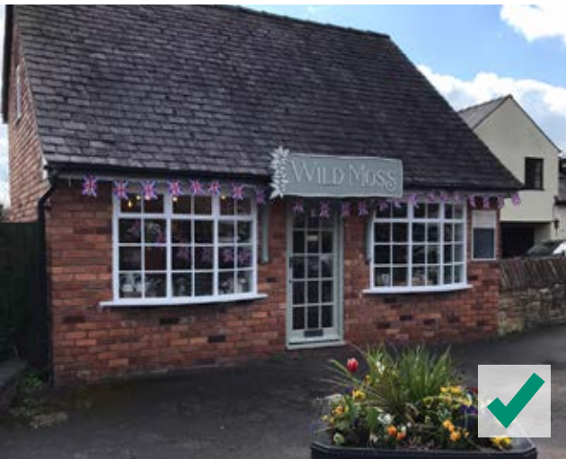
Figure 58: Sensitive and historic context driven commercial frontage on High Street
