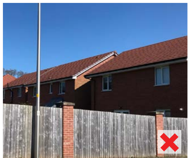
Figure 53: Generic design where there is little architectural detailing or reference to local character should be avoided.
