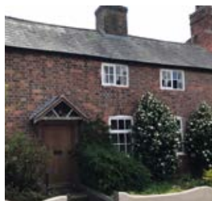
Timber frame pitched / gable overdoor canopy
