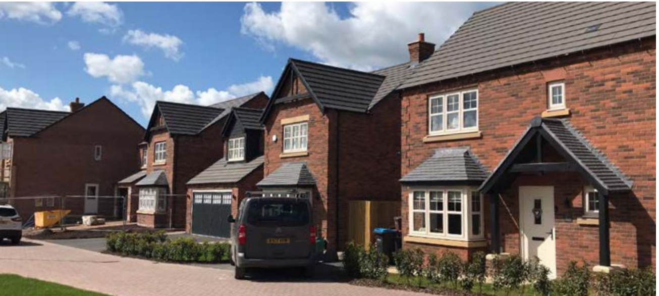
Figure 11: High quality design reflected by mix of facade detailing and materiality.
