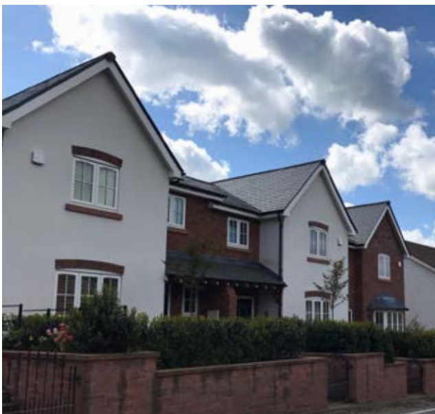
Figure 37: Terraces fronting Wrexham Road.
