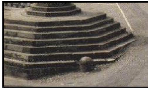
(L) Aerial view of the castle motte which contains the redundant reservoir (R) The metal dome by The Cross which covers a valve which was part of the piped water system.
